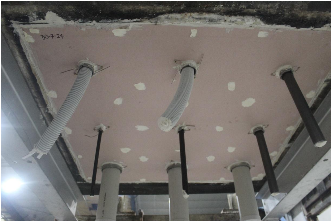
Figure 1 – Exposed face prior to test commencement
